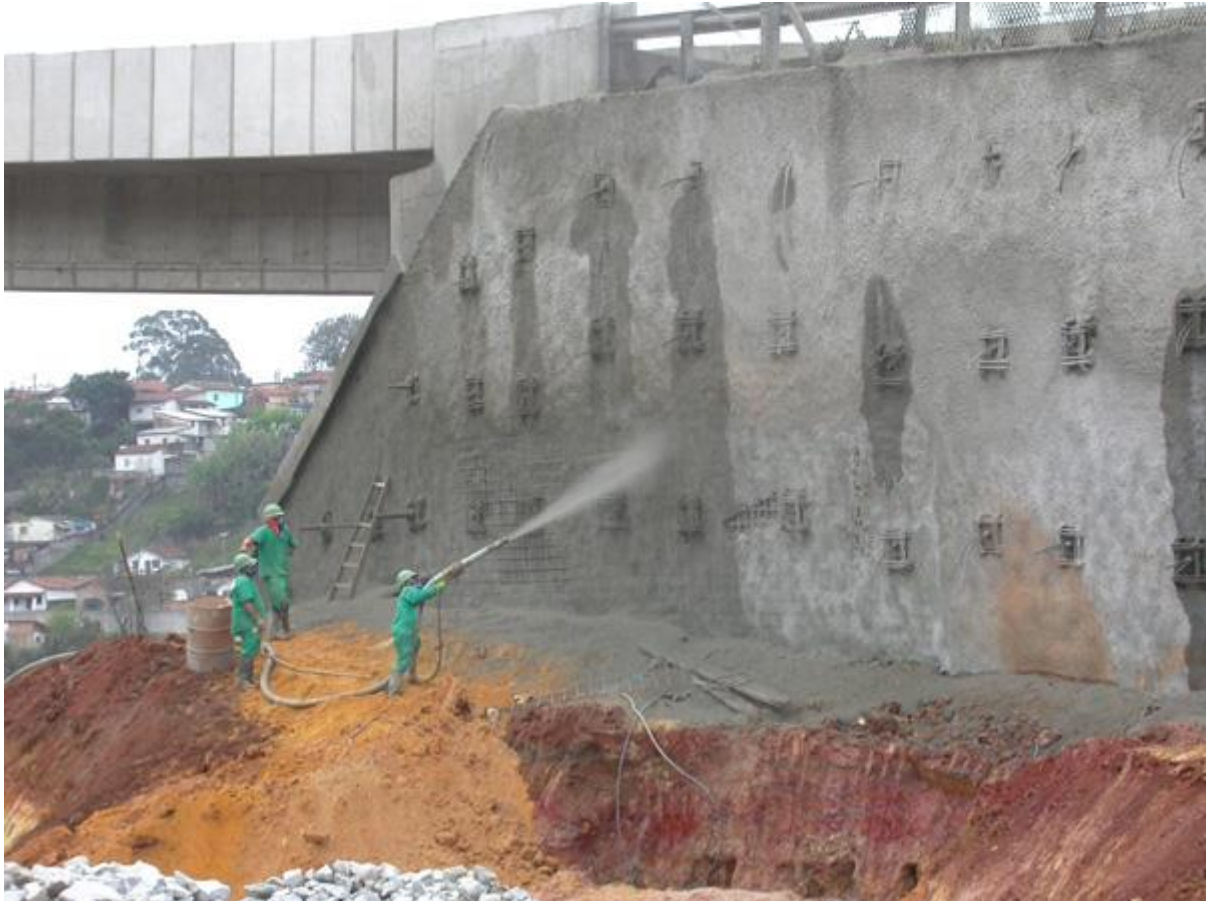
Figura 20 – Solo grampeado (soil nailing)
