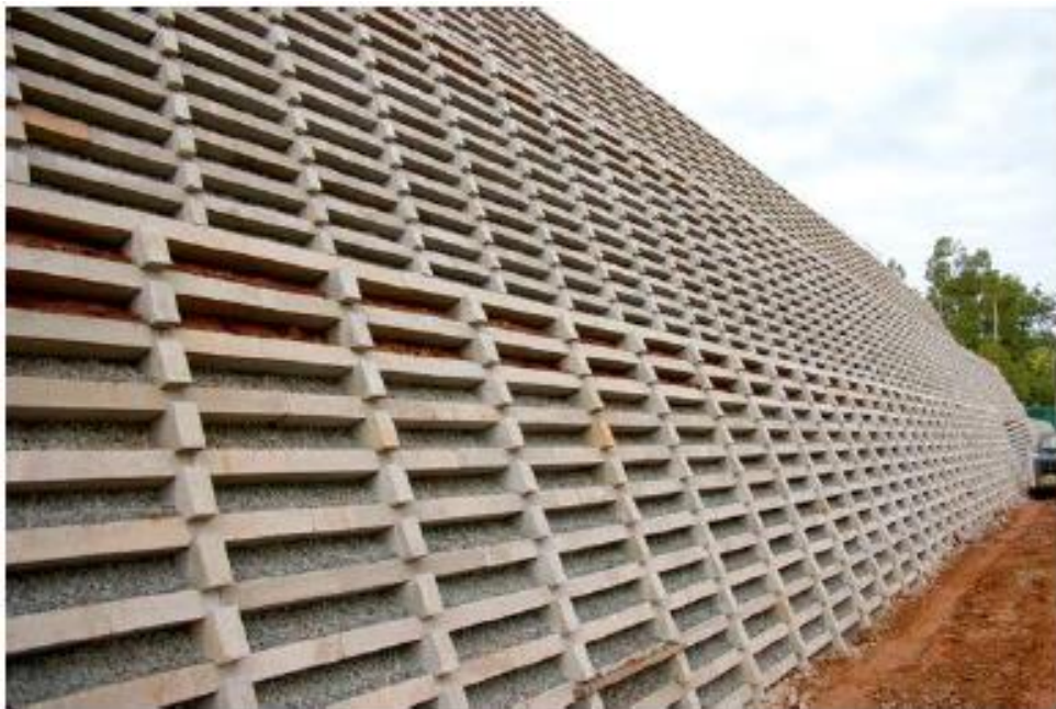
Figura 7 – Crib-wall
