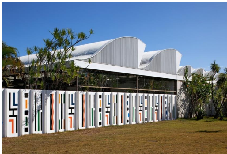
Figura 50 - Fachada do Hospital Sarah Kubitscheck
