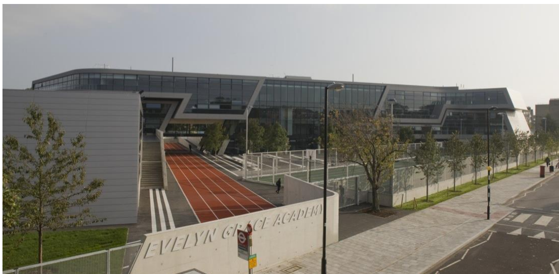
Figura 16 - Evelyn Grace Academy – Vista Fachada Principal
