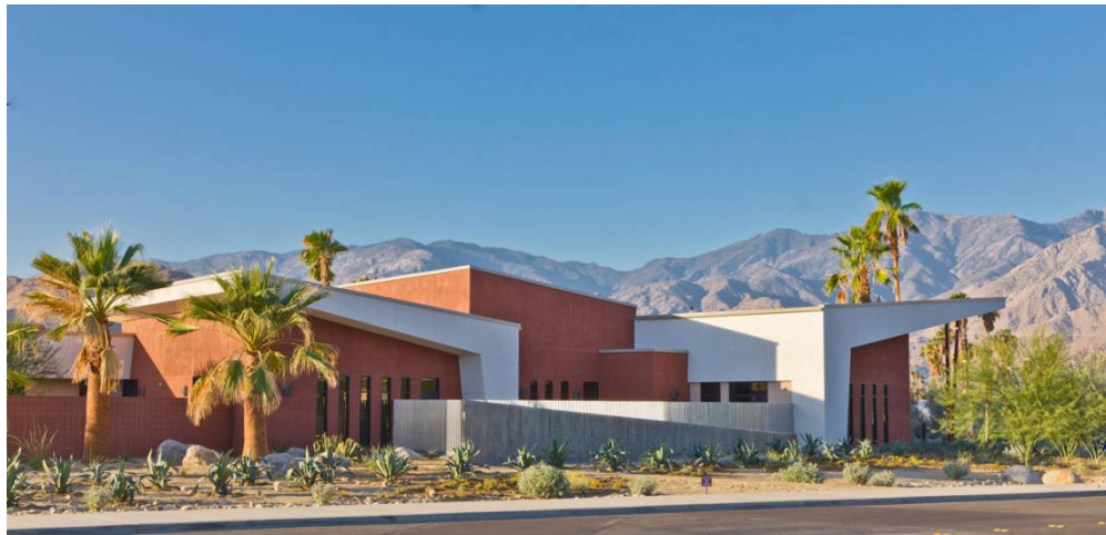
Figura 30 – Vista Lateral Palm Springs Animal care facility
