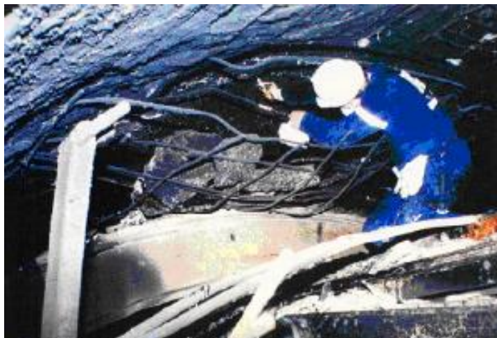
FIGURA 14 - Tunel Great Belt (1994)
