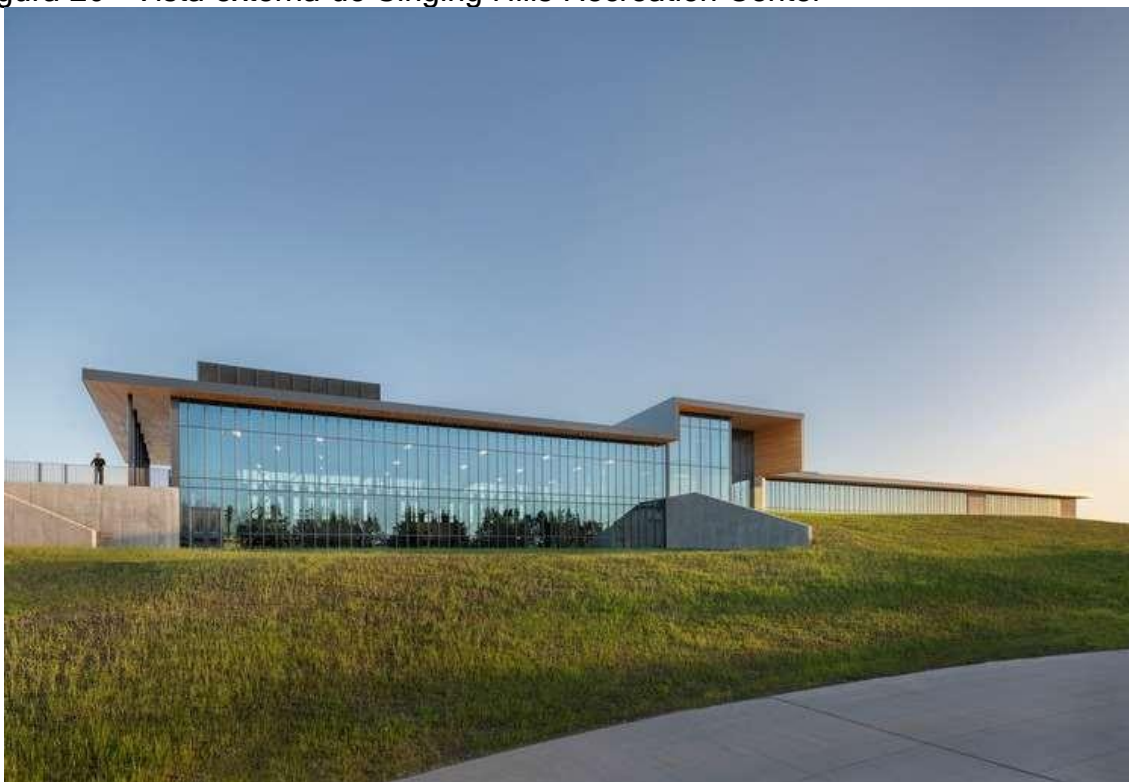
Figura 20 - Vista externa do Singing Hills Recreation Center
